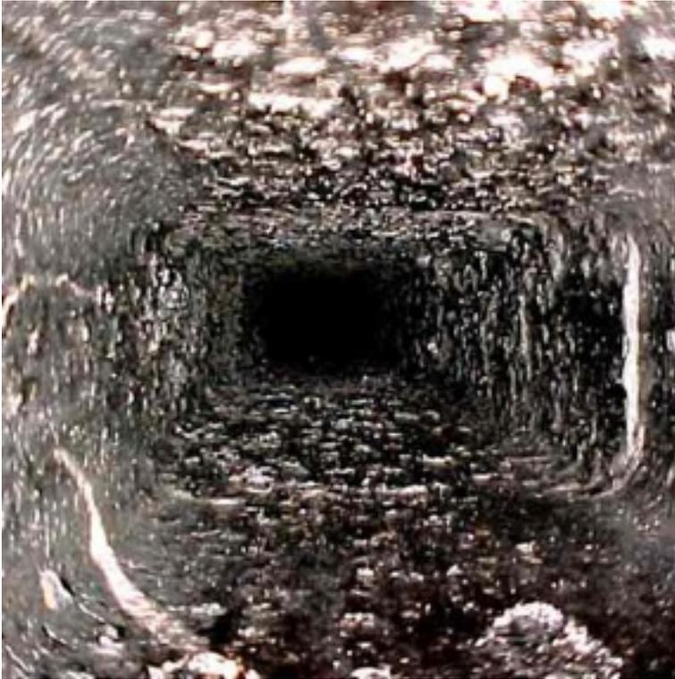
Third degree creosote buildup is the worst of them all. This occurs when the flue temperatures are low and/or combustion is incomplete. This is common when any of, or a combination of, these conditions exist:
